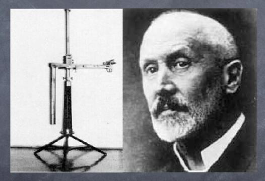
tested Equivalence Principle with torsion balance to 5 parts in a billion
